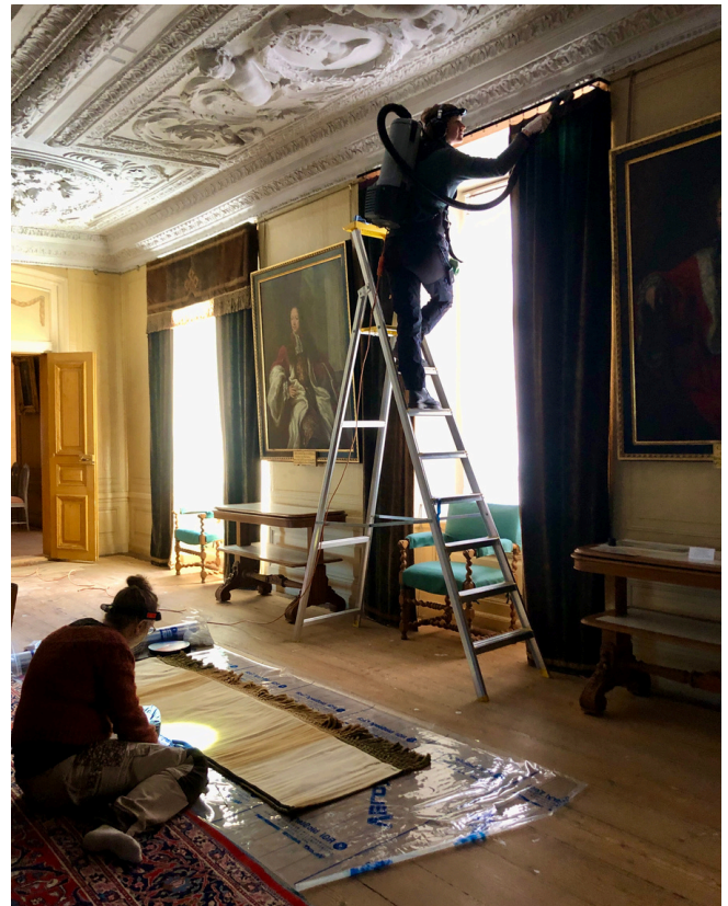
Housekeeping and doing emergency repairs at a castle. Copyright Nationalmuseum Sweden
