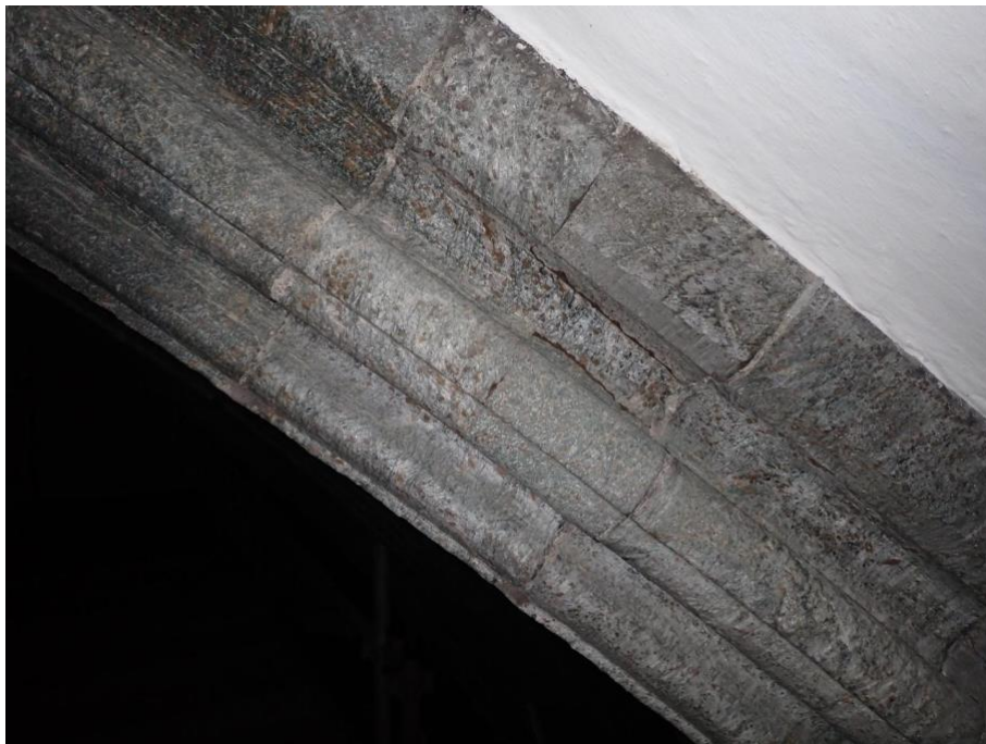
Figure 3: Medieval stone indents attached with adhesive.
