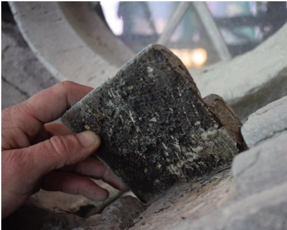
Figure 2: Historic adhesive repair on Stavanger cathedral. Image: © B. Ebert, Museum of Archaeology, University of Stavanger.
