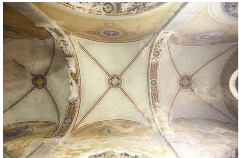
Figure 6 The nave’s vaults
