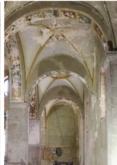
Figure 8 The northern aisle
