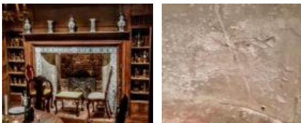
Figure 14: (Left) Vauxhall Fireplace (1969.4722.002-036) was damaged by a flood in 1987; (right) delaminating plaster surrounds on Vauxhall fireplace, proper left side.
